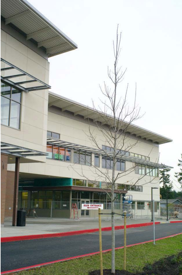
An entry portal and breezeway defines the entry into Campus.
