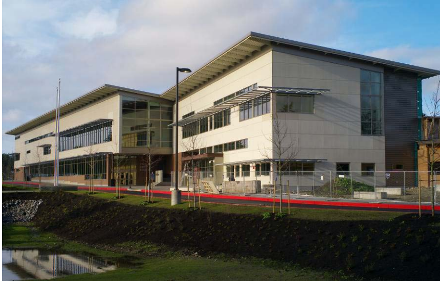
The yet to be painted Classroom and Administration wing of the Student Union Building/Parker Hall Addition to Oak Harbor High School.
